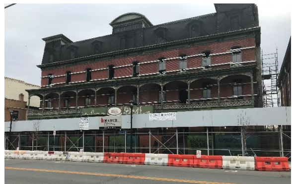
Construction underway, photo D. Reading
